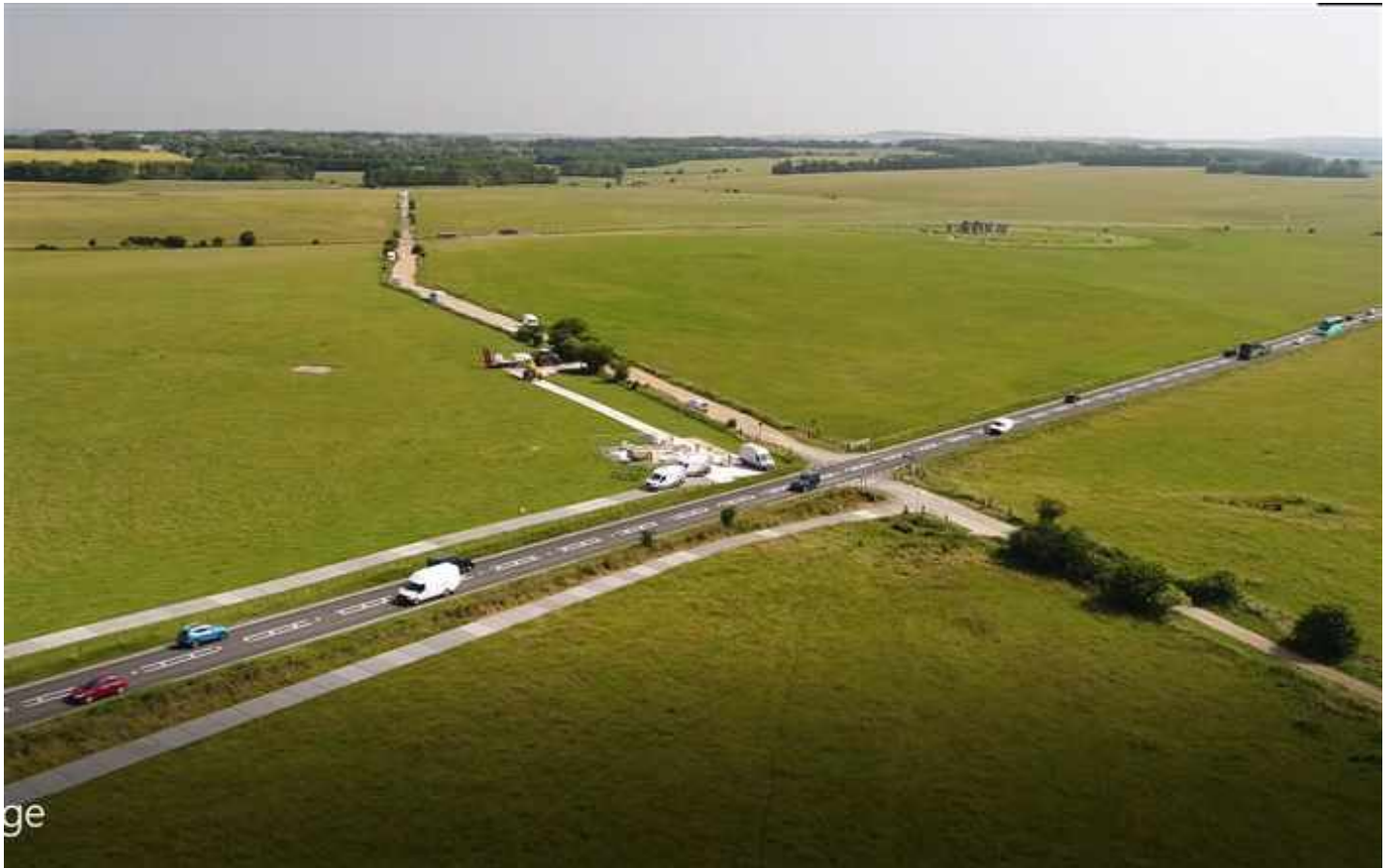
Aerial view over R71903 looking north east
